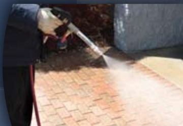
De-ice confined areas with hand spray wand
